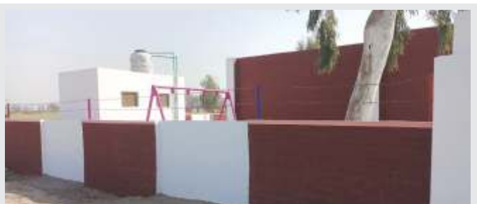
Government Primary School Mud Moulvi After Civil Work
