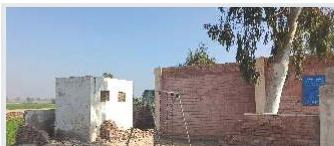
Government Primary School Mud Moulvi Before Civil Work
