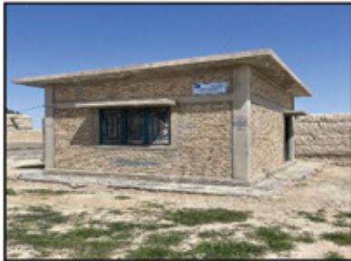
DWSS pumphouse constructed under BRACE Programme in Qilla Askan Khan UC
