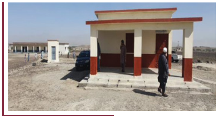
Figure 44 Construction of Water Tank in School Building in UC Sammi, Kech
