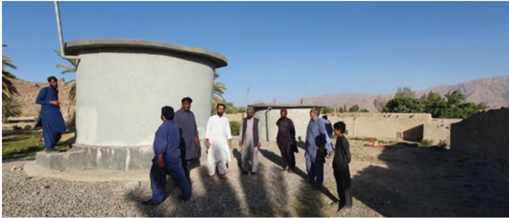
Scheme: Drinking Water Supply Visit at UC Balina Wahir, District Khuzdar, Balochistan
