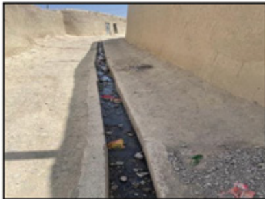
Drainage System Constructed under BRACE Programme in Manzaki UC, Pishin
