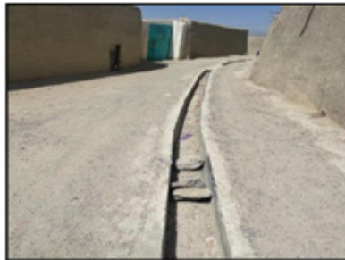
Drainage System Constructed under BRACE Programme in Manzaki UC, Pishin District
