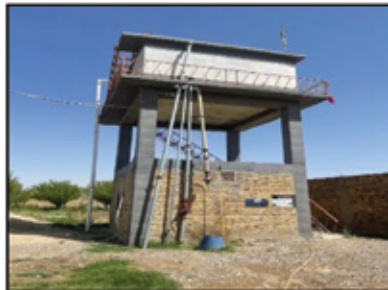
Overhead Surface Tank Constructed under BRACE Programme in UC Yaro 2
