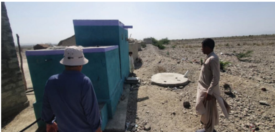
Scheme: Rehabilitation of Government Services (Communal Toilet) Site visit, UC Solband, District Kech, Balochistan
