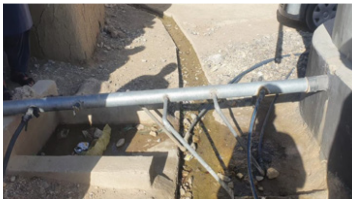
Figure 50 Extension in Pipes by the Community
