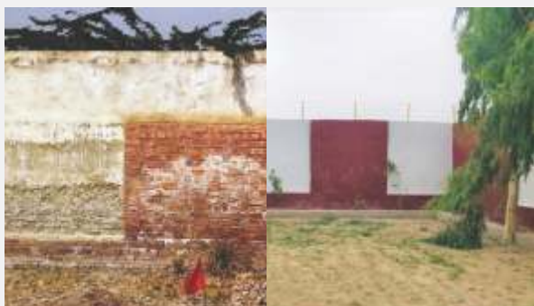
Condition of School Boundry Wall after Completion of Civil Works
