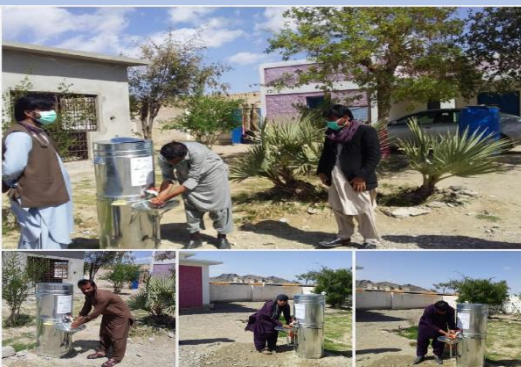
Installation of Handwashing Unit, district Washuk
