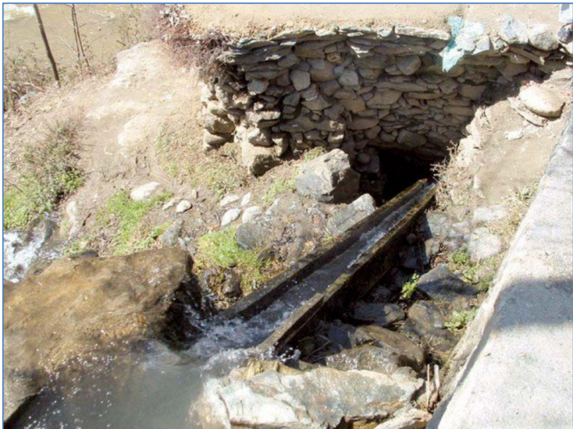
Figure 27: Channel constructed for transferring water to stone mill for grinding of wheat and corn in Kalasha Valley, Chitral
