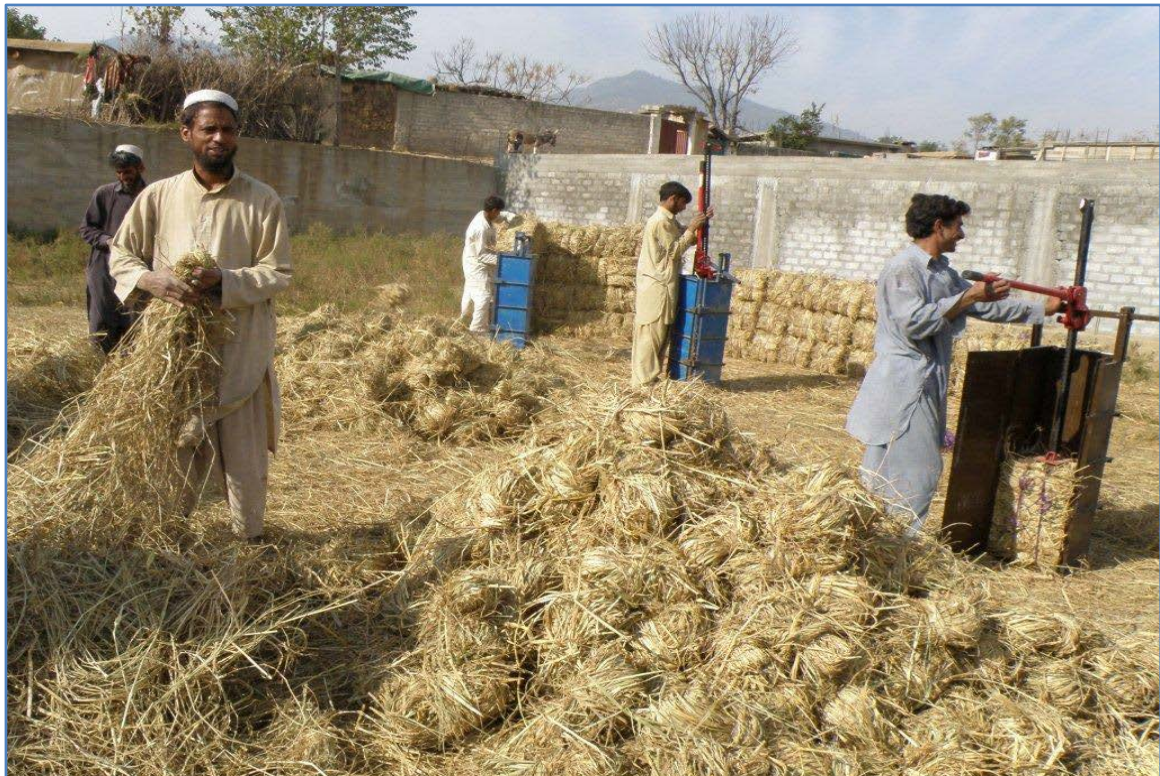
Figure 26: Construction steps of straw bale house for earthquake proof (Courtesy: Green Prophet)
