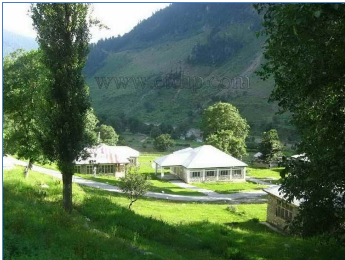
Figure 34: Corrugated galvanized iron sheets used for roof
