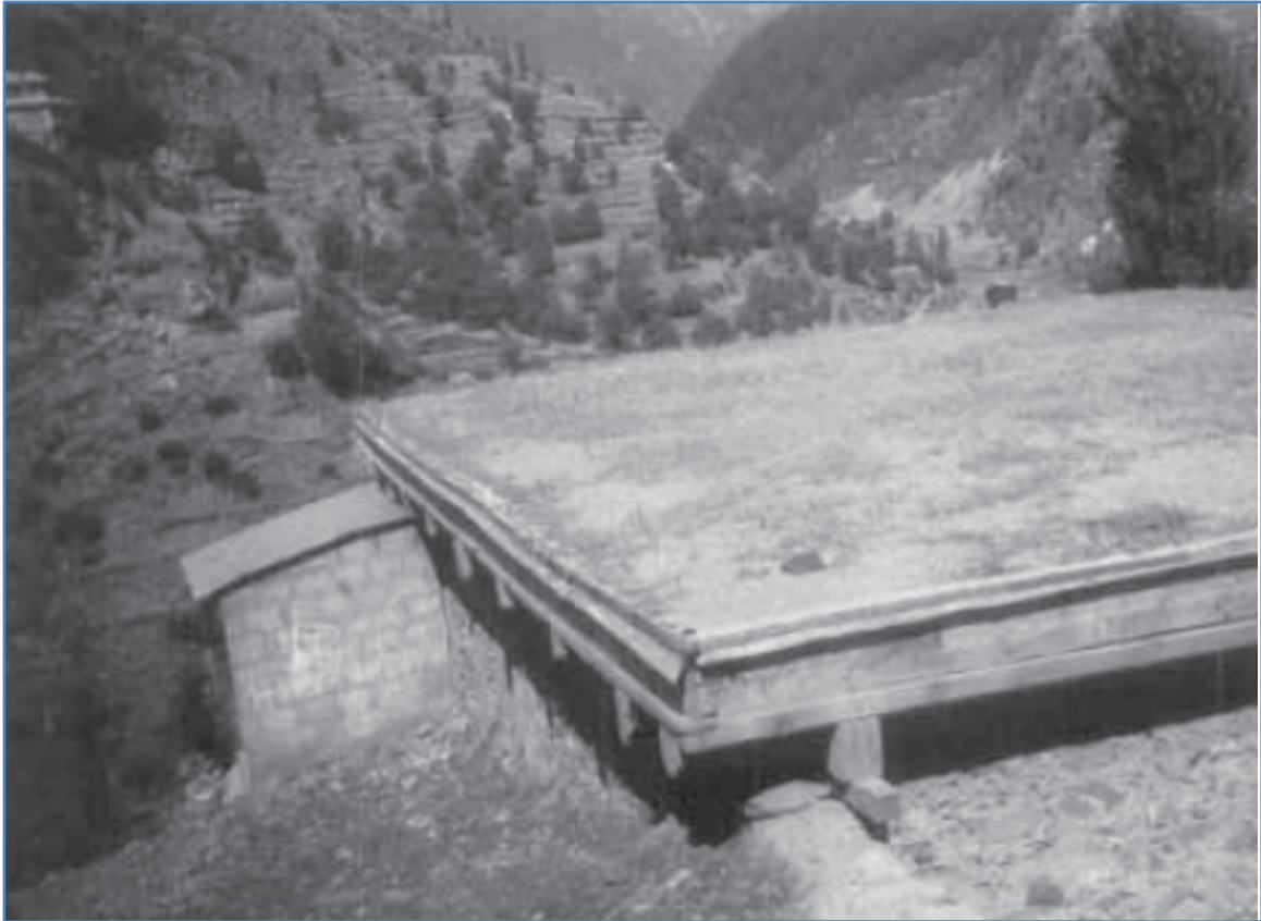
Figure 33: Roof technique to prevent seepage
