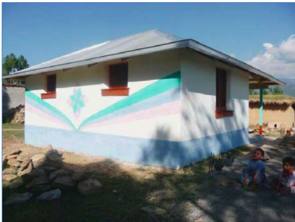
Figure 23: Clay-plaster reinforced, a fabricated straw bale house costs half the expenses of modern building for every square foot
