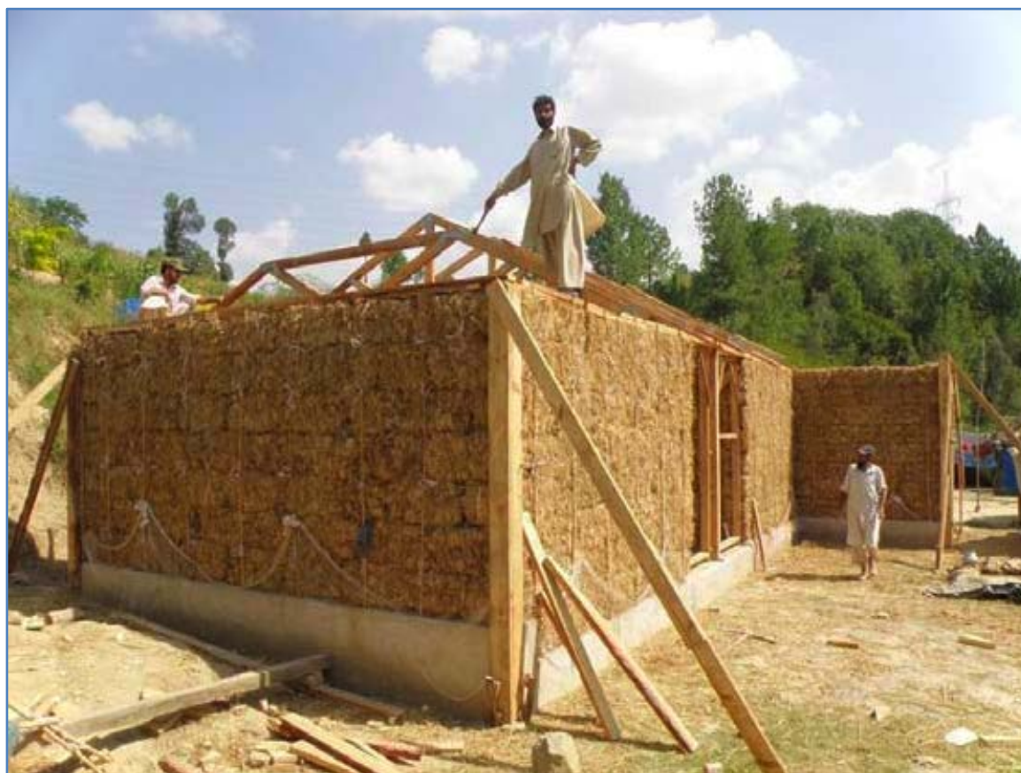
Figure 22: Twice as energy efficient as a conventional house, straw bale makes for environmentally friendly earthquake-proof homes
