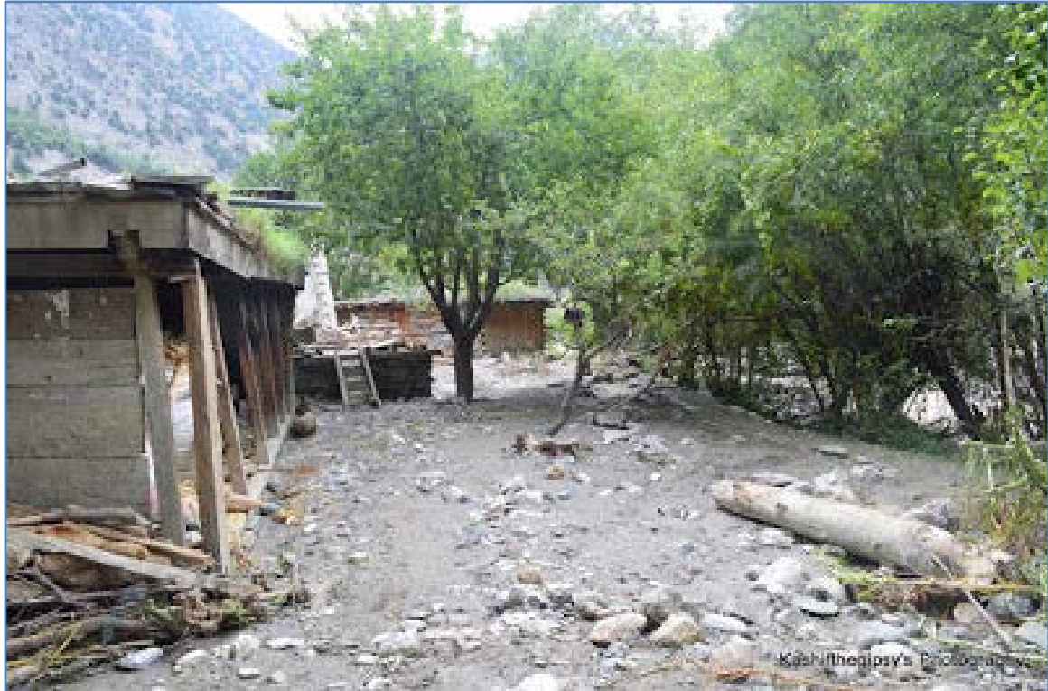
Figure 38: Flood struck homes (Palarog Village, Rumbor Valley)
