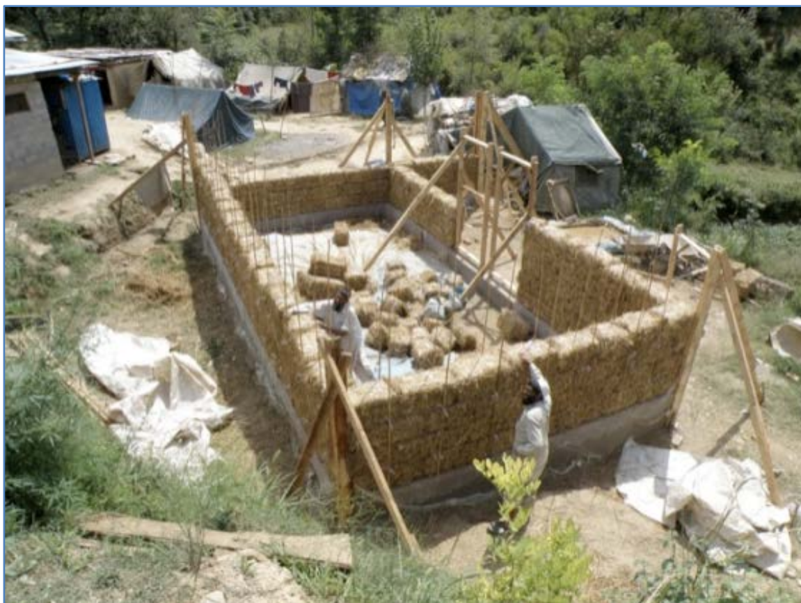
Figure 25: Tightly packed walls and a gravel weighted foundation creates better weather-proofing
