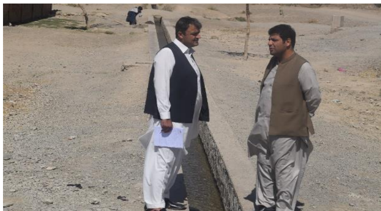
Irrigation channel constructed by BRSP in UC Daman Miralzai Chaman
