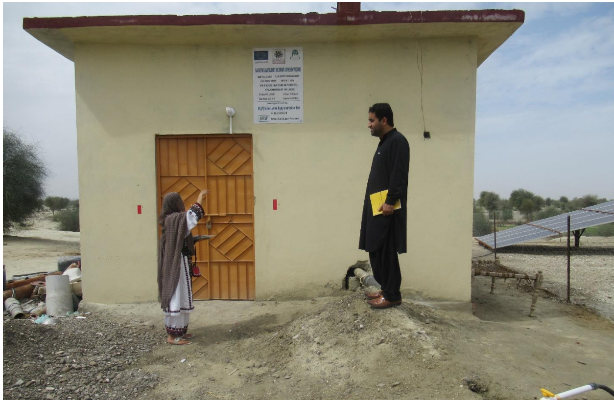
Water Supply constructed under BRACE Programme in Kunchiti village
