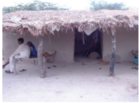
UDMC Kadhan rebuilt the house affected by fire at settlement Jhummon Bhangoro, district Badin.
