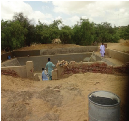
Rehabilitation of rain water harvesting pond at revenue village Vjiheto, district Tharparkar helped in reducing vulnerabilities of residing communities during drought situations.
