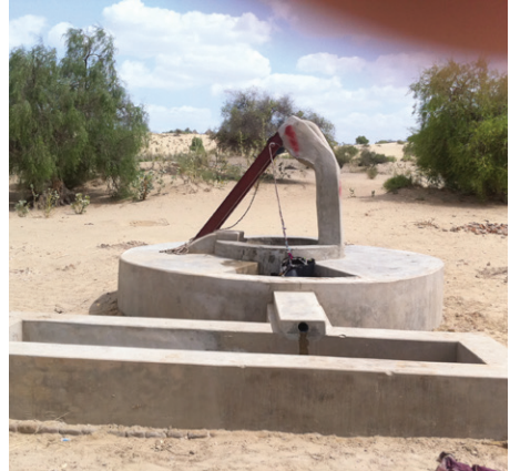
The rehabilitated dug well in VDMC Moharano is source of water close to the settlements.
