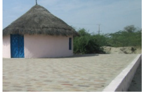
The Rescue Point built during Phase-I provided shelter to fire affected household in VDMC Saddori Sar.
