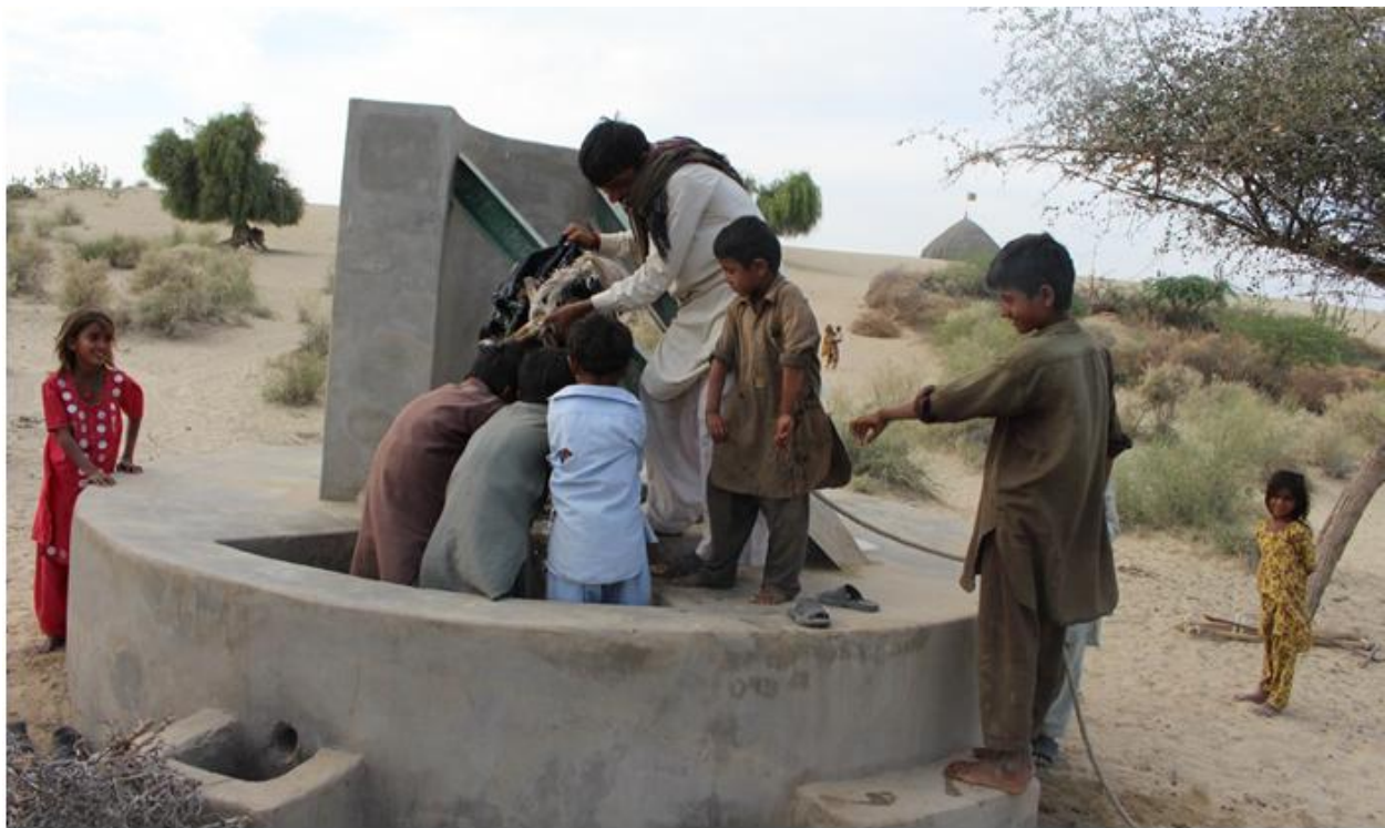
To mitigate drought at district tharparkar the project supported financially VDMC members in rehabilitation Water Related Infrastructures. Dug well is one such type of WRI rehabilitated under the Tahafuz project.
