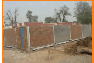
Figure 23: Constructed boundary wall around the school
