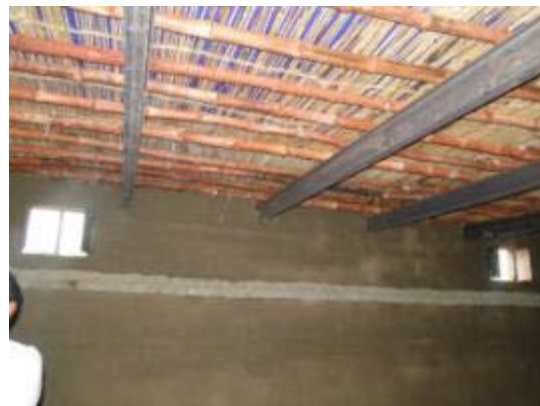
Inside view of Mud TS
