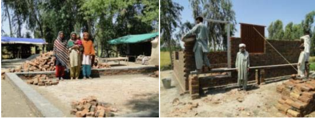
District Mianwali: Under Construction Transitional Shelter
