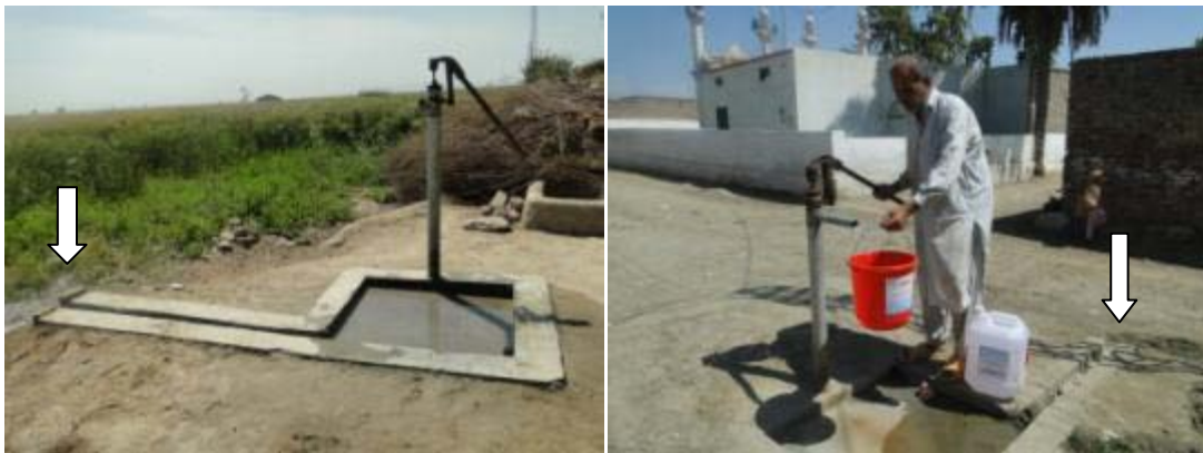
District Mianwali: Hand pumps with improper outlets
