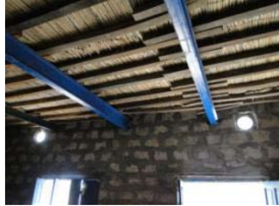
Inside view of Cemented Block TS
