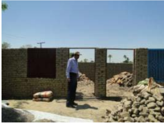
Rajanpur: Sharing of Walls
