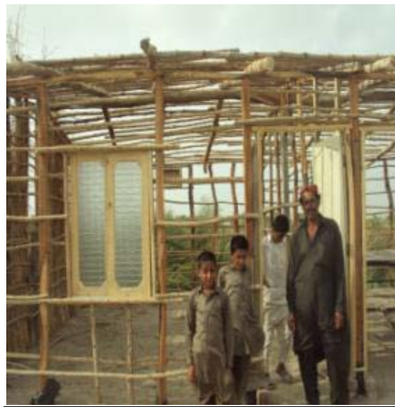
Beneficiaries with under construction Transitional shelter
