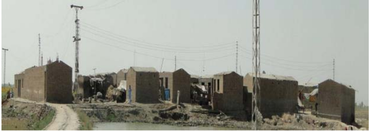
Beautiful One Room Shelters by USAID Bahaal in the village of Laandi Ali Murad Shah
