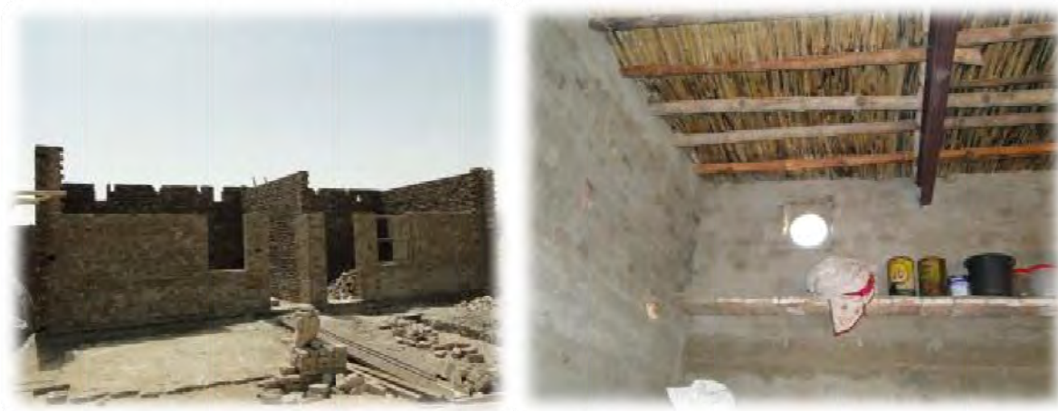
SGA Transitional Shelters during different stages of construction
