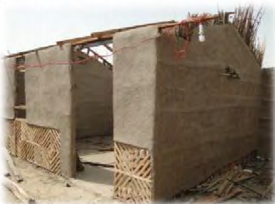
Wooden Transitional Shelters in the district of Thatta, during different stages of construction
