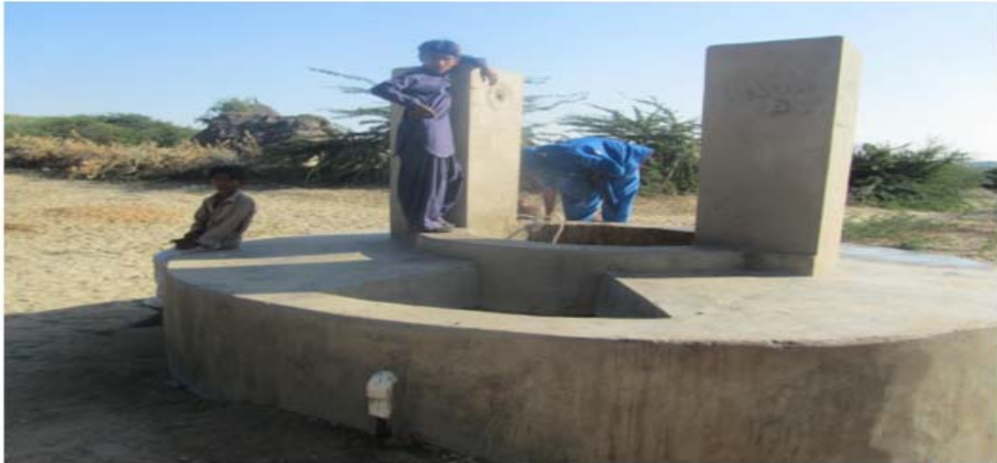
Women fetch water from dug well at UDMC Mohrano District Tharparkar. This well previously un lined is now rehabilitated with Brick masonry.
