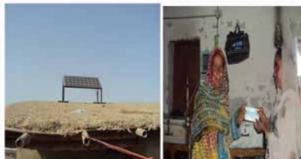
Solar Electrification System
