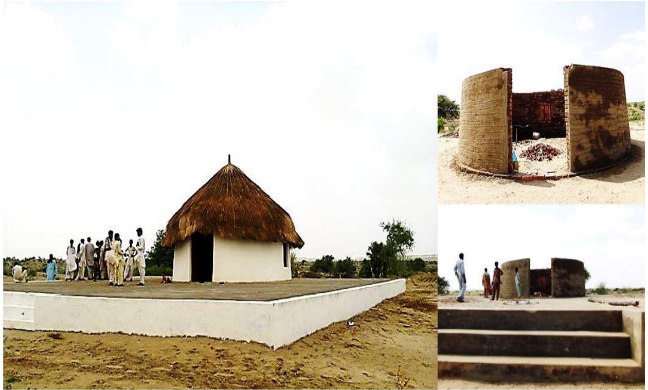
Construction of a Rescue Point VDMC Wingi, Union Council Jhirmiryo, District Tharparkar
