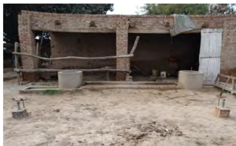
2 Biogas Plants (15M 3 each) constructed in Haji Irshad's Farm House
