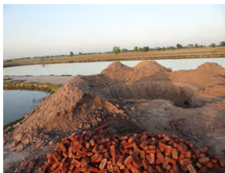
A new 20m 3 Biogas Plant under Construction at Walayat's Fish Farms
