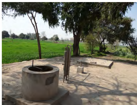
Biogas Plant constructed in Mirza Manzoor's Farms
