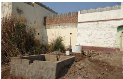
Muhammad Nawaz BCC Constructing 3 new Biogas Plants in Chak 4997-JB
