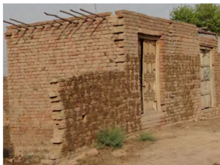
The Wall Was Used To Make Dung Cakes before the Biogas Facility
