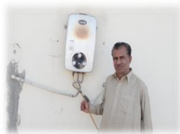
Mr. Tariq using water geeper on Biogas Plant
