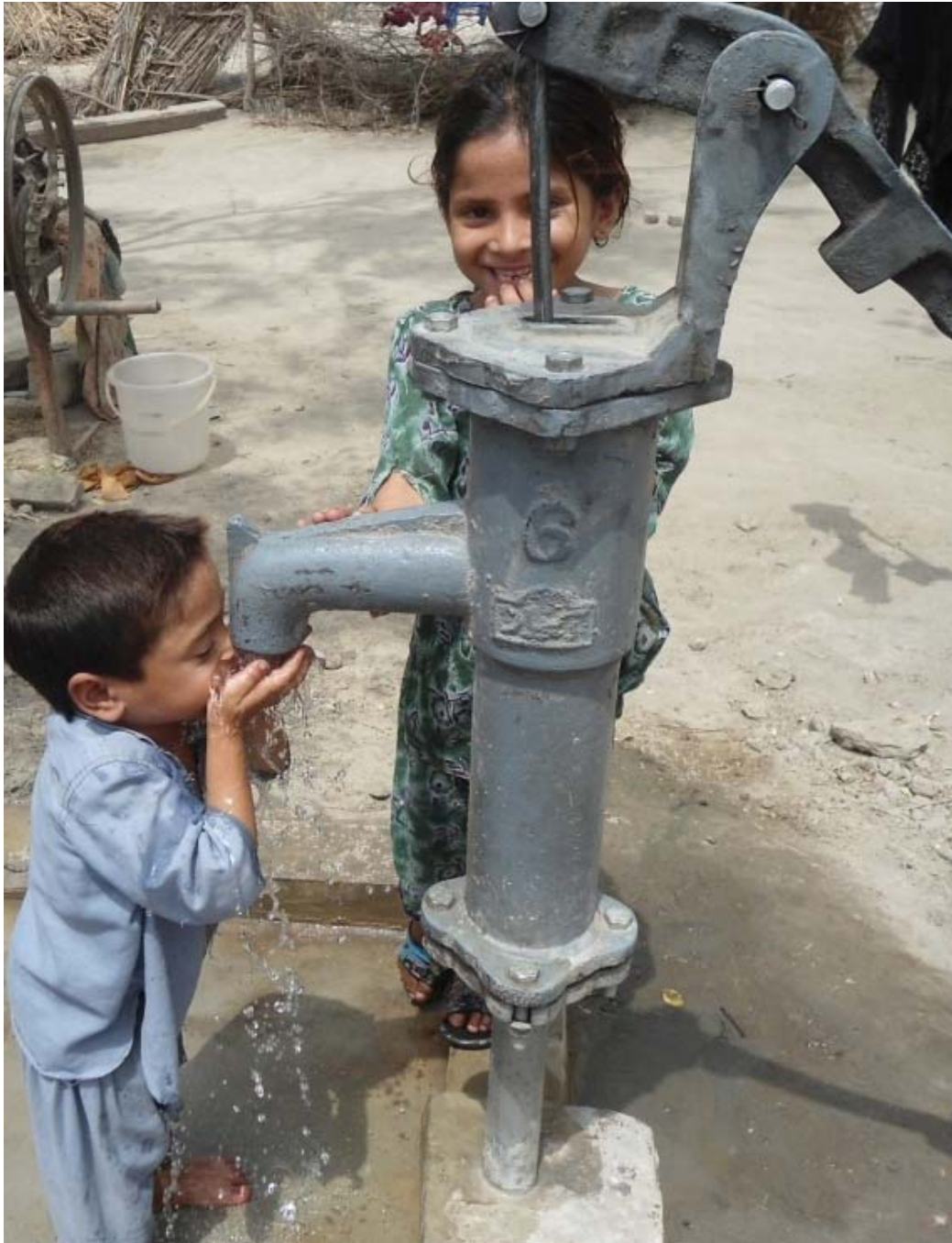
Handpumps were an essential feature of the multisector assistance by SRSO
