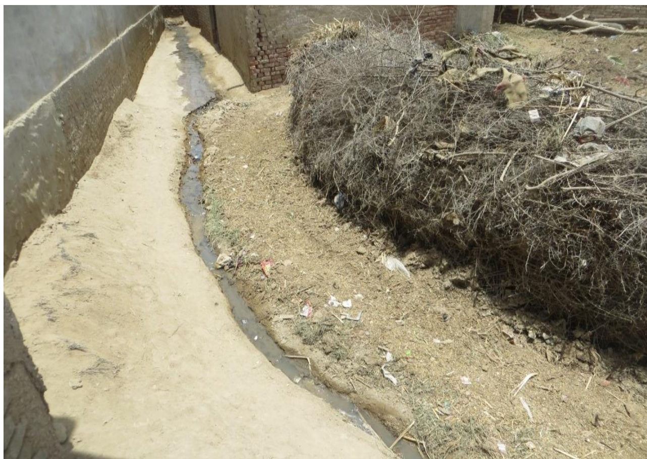
Figure 7: Street lacks the proper planning in the villages of UC Masoo Bozdar
